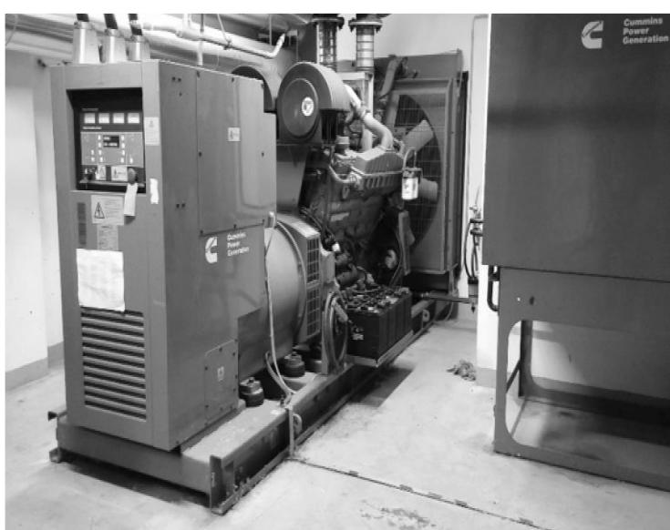
The particle filter installed in front of the fuel injector of the generators filters out impurities and eliminates the resulting malfunctions. In the event of a complete power outage, the generators start automatically within 30 seconds to signal uninterrupted systems.
